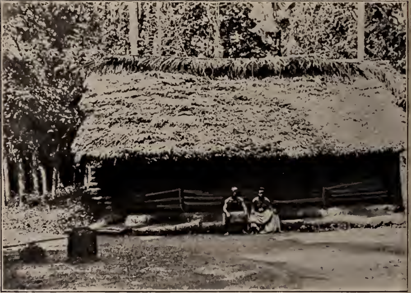
The Iko pillar before the native court house at EBİYAWMALO. See page 195
